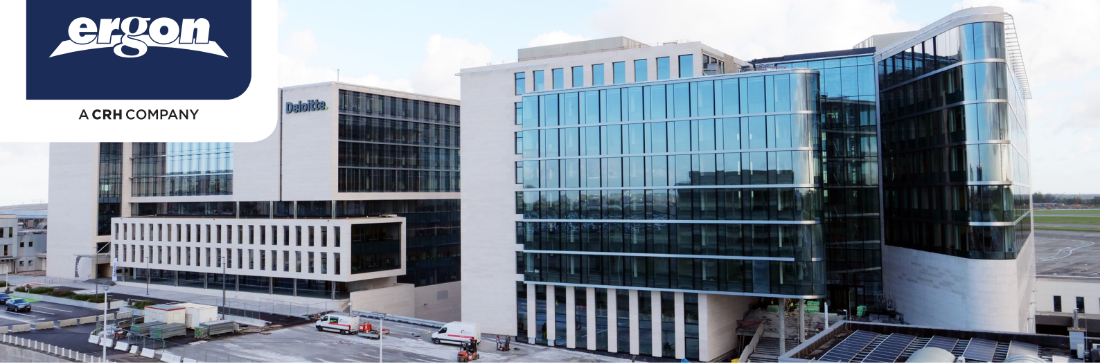
Project "Gateway" in Zaventem
